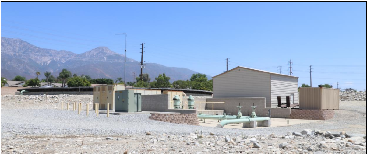
Photo 3: Water reservoir behind (north of) modern building and equipment, view northeast (8/6/24).
