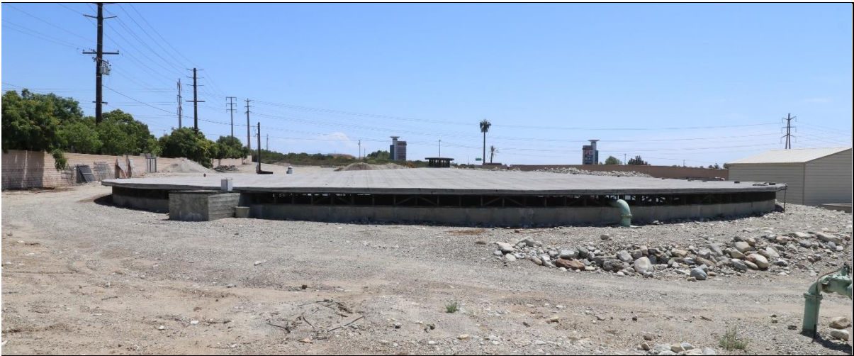
Photo 1: Water reservoir, view east (8/6/24).
